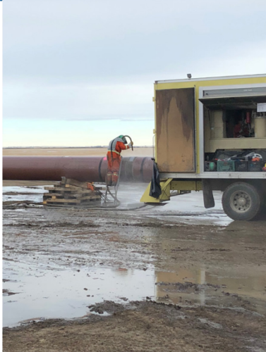
19. Sandblasting – km177+812 – Dec 15, 2017
