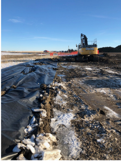
1. Excavator with filter cloth laid in – SF 88 – Dec 11, 2017
