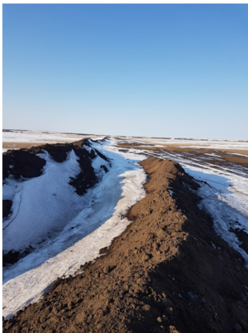
11. Top piles - 145km+900 – Dec 13, 2017
