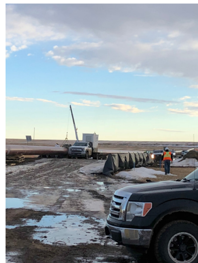
18. Pre heat truck (coating crew) – km177+812 – Dec 15, 2017
