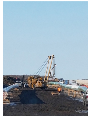
12. Boring Crew - 144km+200 – Dec 13, 2017
