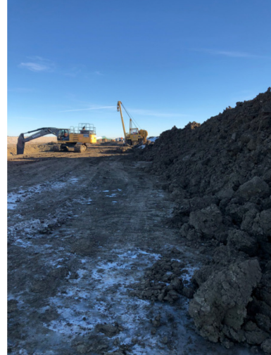
2. Excavator stock piling spill from auger – SF 88 – Dec 11, 2017
