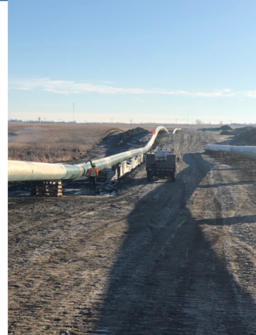
14. 4 man coating crew – km165+700 – Dec 14, 2017
