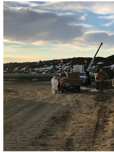
10. Coating crew - Km169+455 - Dec 12, 2017
