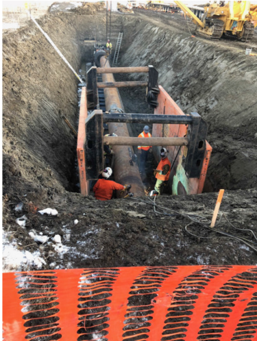
3. Bore crew and welders installing augers– Dec 11, 2017
